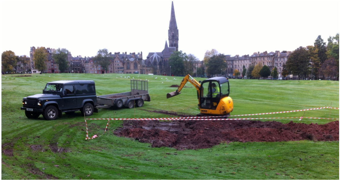
Drainage works on the Links, December 2012
